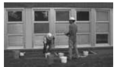
(left) Workers put the final touches on the renovations to the sports event field. (right) Every window on the building was replaced with new energy efficient windows and blinds.
